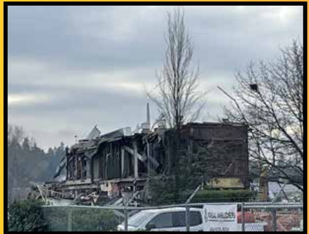
Below: 45 years later, demolition under way.
